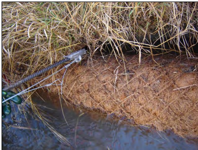
Figure 13. Anchoring coir log in place using Duckbill earth anchors.
