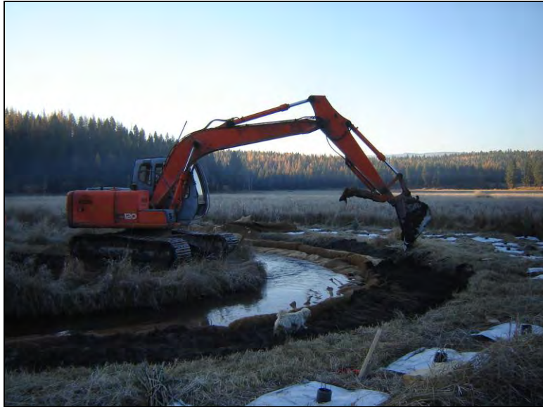
Figure 7. Soil lift 2 during construction.
