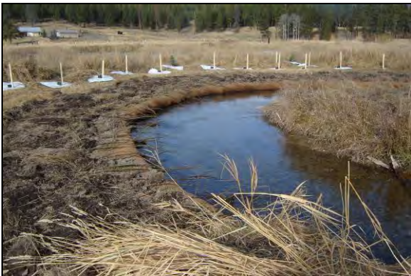
Figure 8. Soil lift 1 (left) and soil lift 2 (right) after construction.
