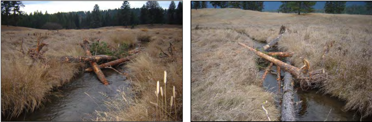
Figure 10. Large woody debris structures #5 (left, looking downstream) and #1 (right, looking downstream).
