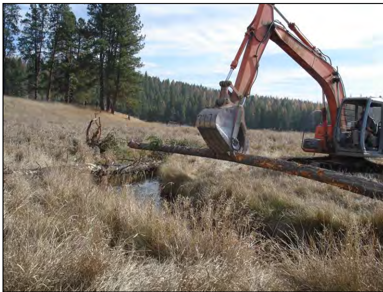
Photo 11. Large woody debris structure during construction.
